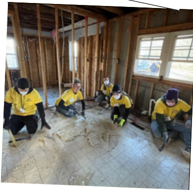
Tearing Up Flooring
